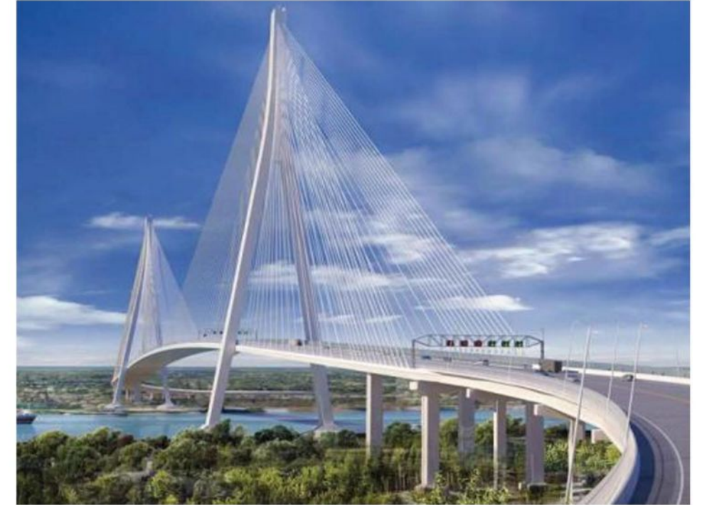
Gordie Howe International Bridge
